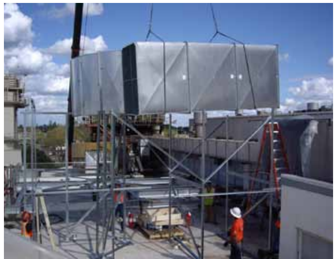
Large duct work is lifted into place
